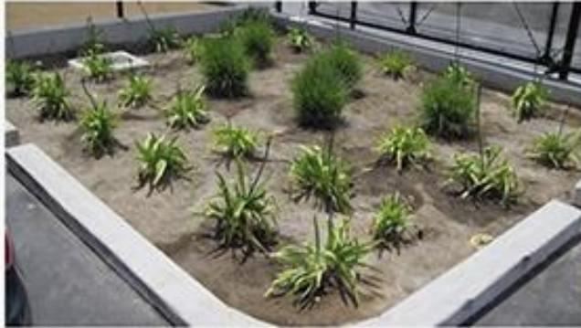
Bioretention Facility: In-ground (Infiltration) planter to ... www.pinterest.com
