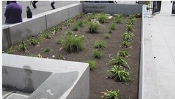
Bioretention Facility: In-ground (Infiltration) planter to ... www.pinterest.com
